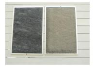
The filter before cleaning on the right is covered in dust.
